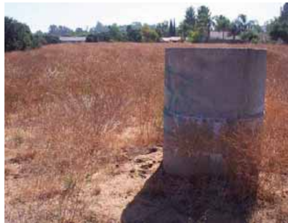
Below: Concrete structure (former irrigation devices) in the western portion of the project site.
